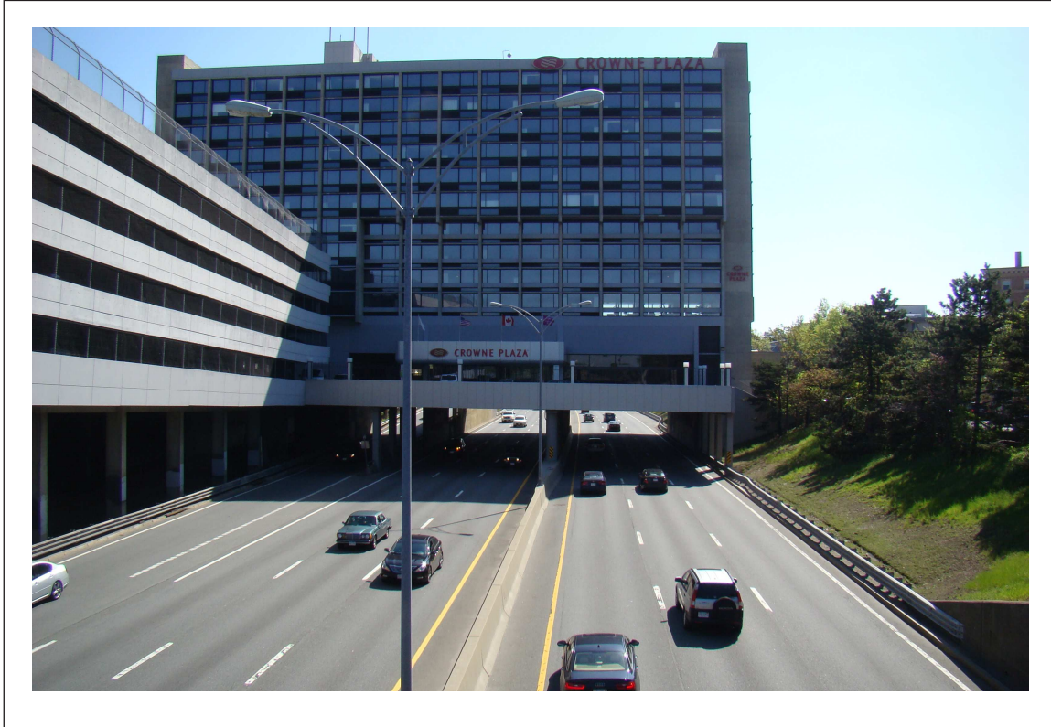
Fig. 12. The Crown Plaza® Boston Newton hotel, built over the Massachusetts Turnpike in Newton, MA
