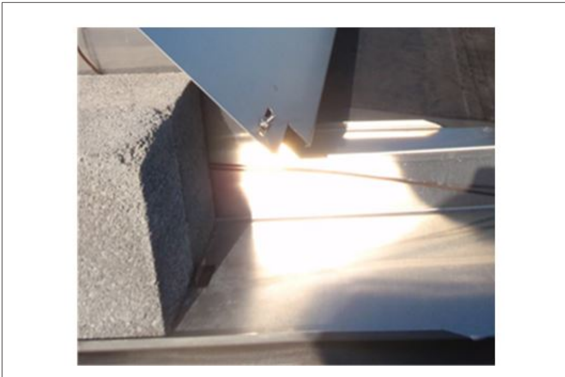
Fig. 2.1.1.11b. Flanged pedestal
