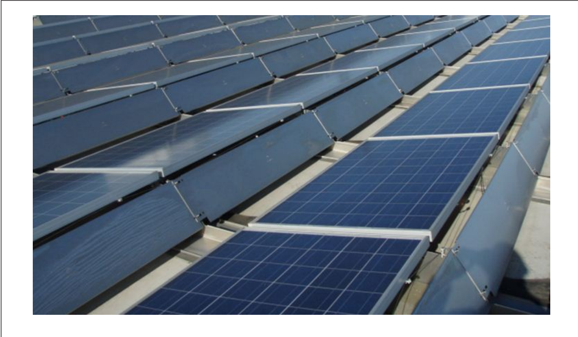
Fig. 2.1.1.1. Wind deflectors provided on the high sides of panels in each row (closed array)
