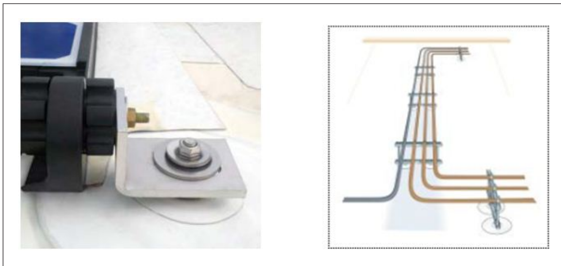
Figs. 2.1.1.9a and 2.1.1.9b. Examples of mechanical anchors used to secure equipment to the roof deck or roof framing
