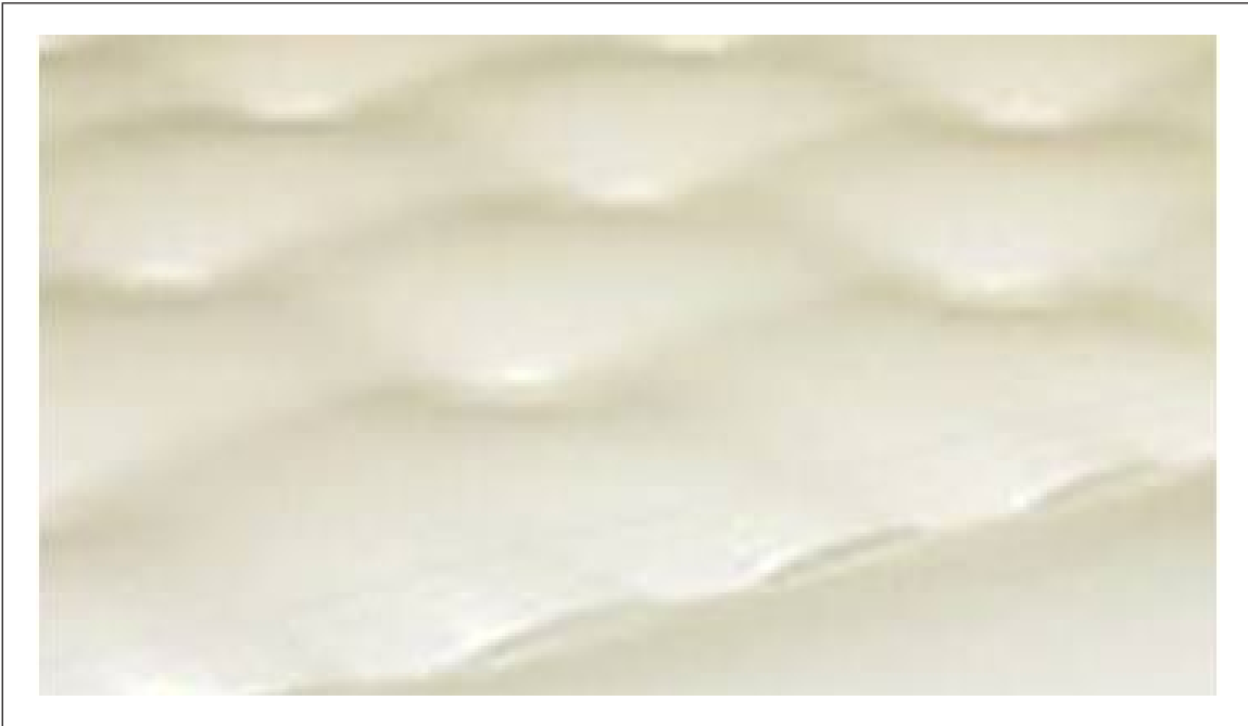
Fig. 3.2.1.1a. Mechanically fastened roof cover billowing when subjected to wind pressure
