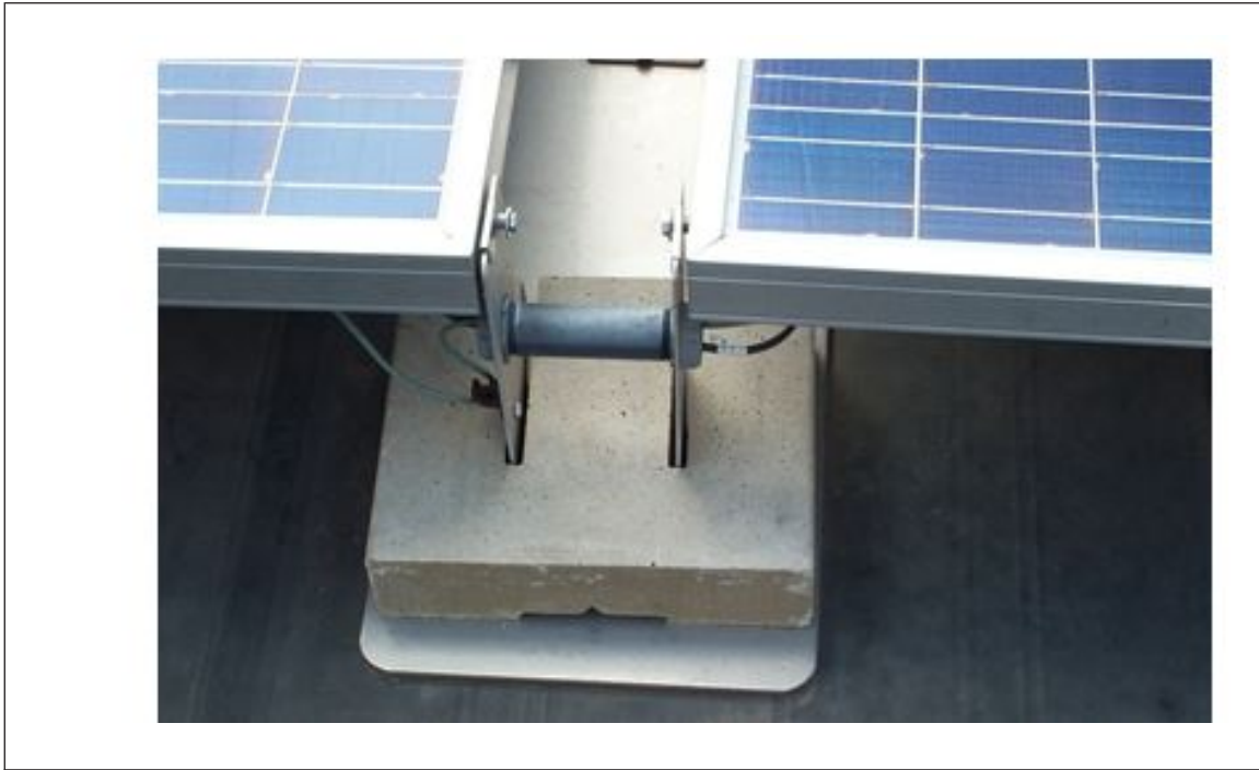
Fig. 2.1.1.11a. Slotted pedestal
