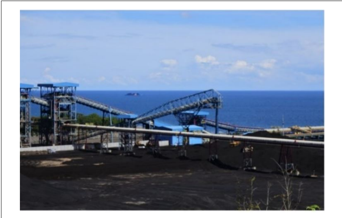
Fig. 3.5.2-2. Example of large open area that could be protected with monitor nozzles
