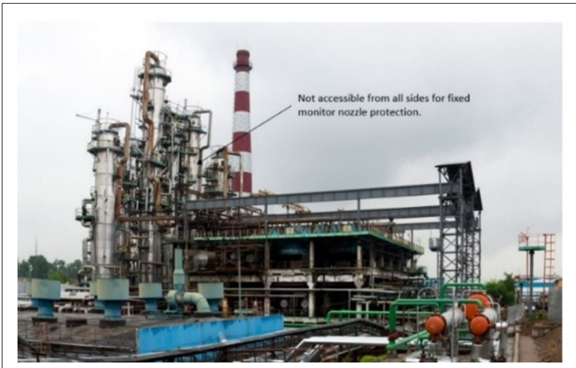
Fig. 3.5.2-5. An object protected by a monitor nozzle must be accessible
