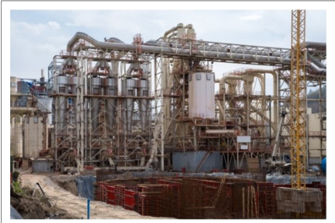
Fig. 3.5.2-4. An object protected by a monitor nozzle must be accessible
