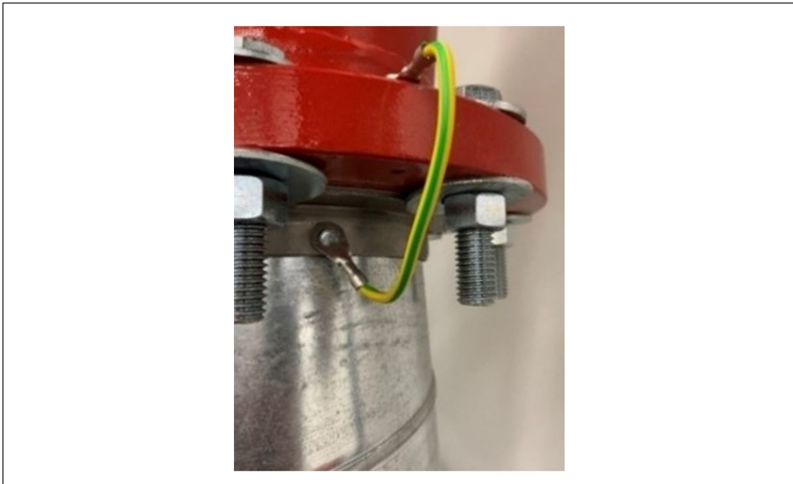
Fig. 2.6.2.1. Bonded metal ductwork
